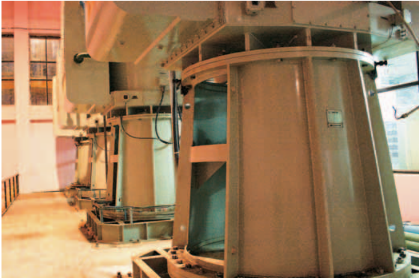
Purandar Lift Irrigation Scheme - Pump Houses with 20 pumps of total capacity 36,700 HP
