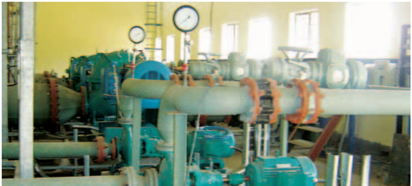
NTPC Sipat Thermal Power Project - Vertical Turbine Pumps of 8500 m 3 /hr. capacity of Make-Up Water System.
