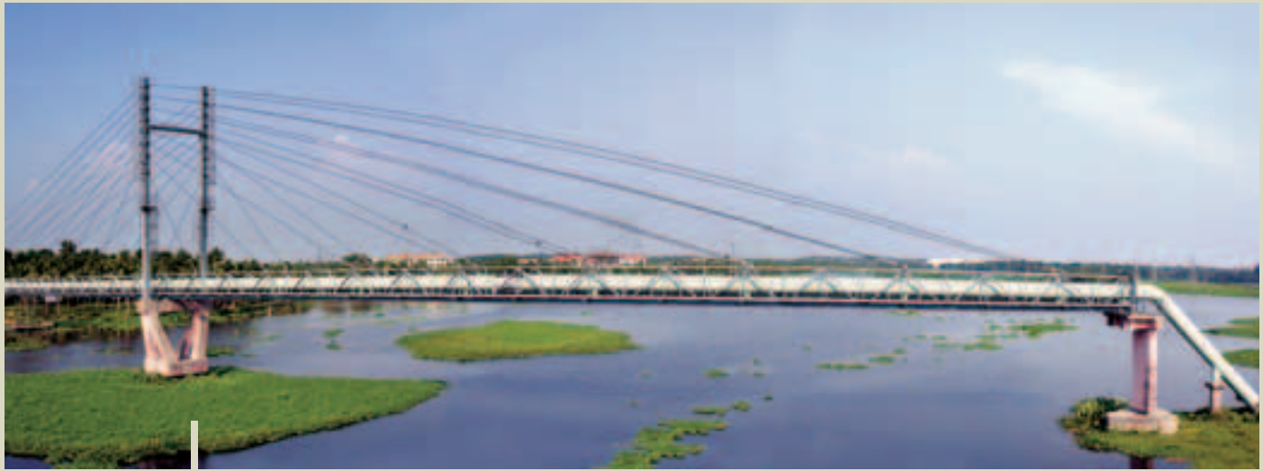
Cable Stay Pipe Bridge for Stand Alone Water Supply Scheme for Kochi Refineries-an EPC Project.
