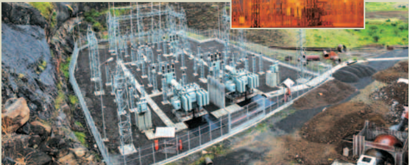
132/33 KV Substation for Purandar Lift Irrigation Scheme.
