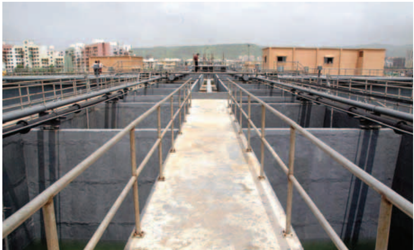
Sewage Treatment Plant based on Sequential Batch Reactor (SBR) Technology for CIDCO Mumbai.
