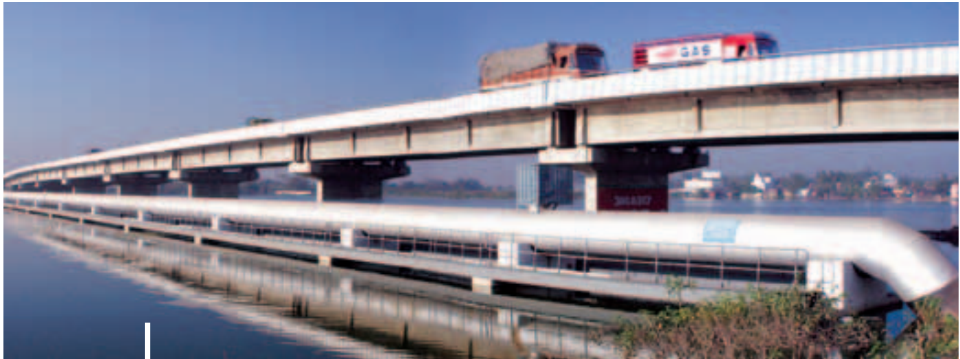
Clear Water Supply Transmission Main-M.S. Pipeline of 1875 mm & 1500 mm dia and total length of 114 kms of Veeranam Water Supply Scheme.
