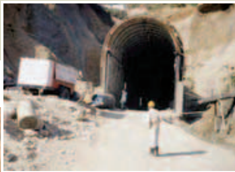
Diameter of the tunnel: 6.5 (width) x 9.5 metres Cross section: 55 square metres
