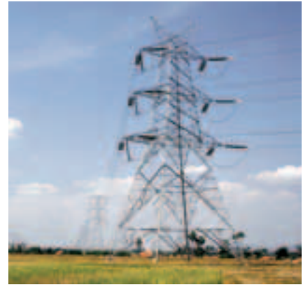
400 KV Double Circuit Transmission Line from Visakhapatnam to Kathipudi – 100 kms in length on EPC basis.
