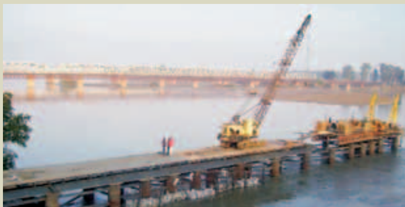
BOT PROJECT – Toll-way bridge on the Jalandhar-Amritsar highway, has 16 piers spanning 0.7 kms, and a total height of 49.34 metres.
