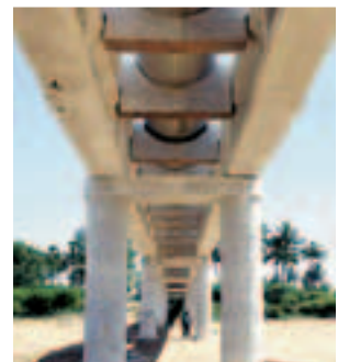
Clear Water Supply Transmission Main-M.S. Pipeline of 1875 mm & 1500 mm dia and total length of 114 kms of Veeranam Water Supply Scheme.
